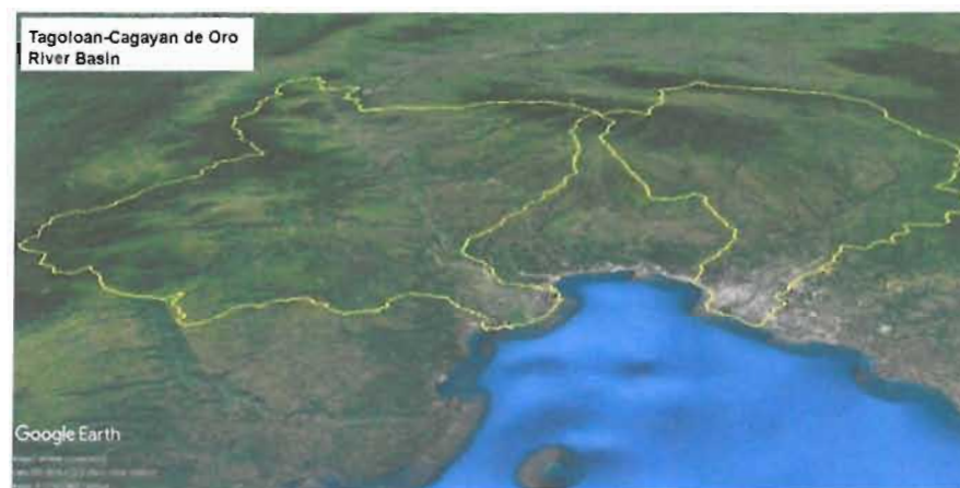
Figure 4. The ridge to reef landscape-seascape of the Cagayan de Oro and Tagoloan Riverbasins showing Macajalar Bay as the outlet of both riverbasins.
